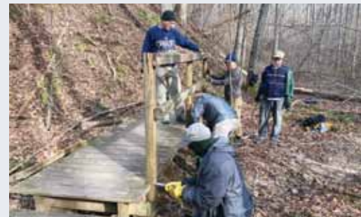
Volunteer Trail Crew members demonstrate their engineering and construction skills in repairing pedestrian bridges along the hiking trail system.
